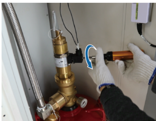
Figure 2-3 Loosening the solenoid valve power plug
