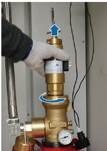
Figure 2-4 Removing the solenoid valve
