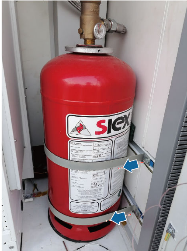
Figure 7-81 Loosening the hose clamp
