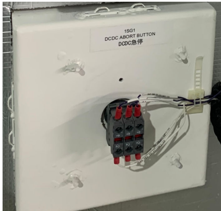
Figure 7-41 Disconnecting cables from the abort button
