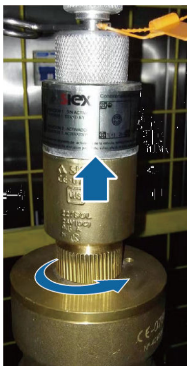
Figure 7-79 Removing the solenoid valve
