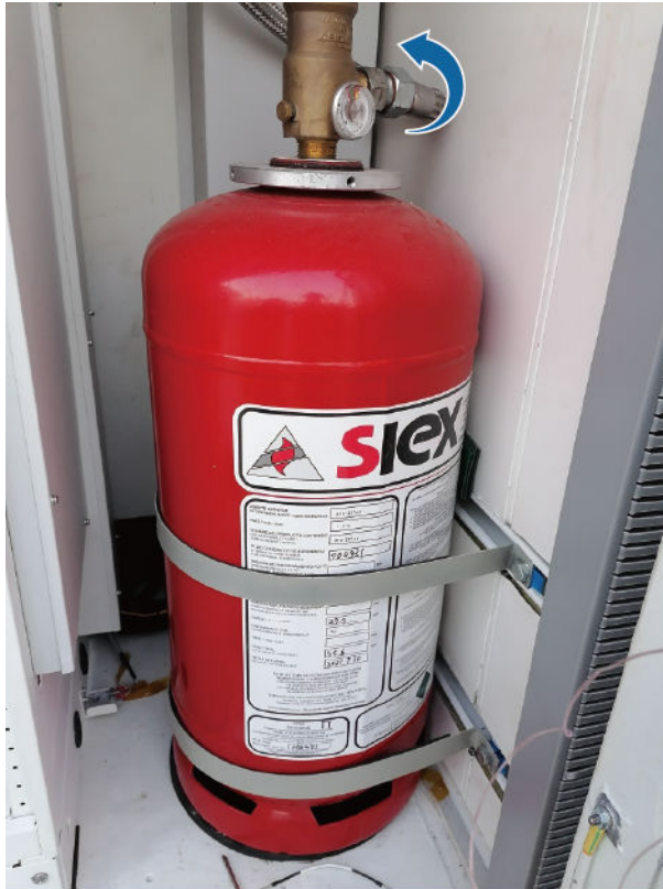
Figure 7-80 Loosening the fire extinguishing high-pressure hose
